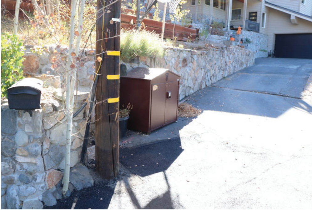
Photo 9: Panned right from previous photograph. View of neighbor's retaining wall.
