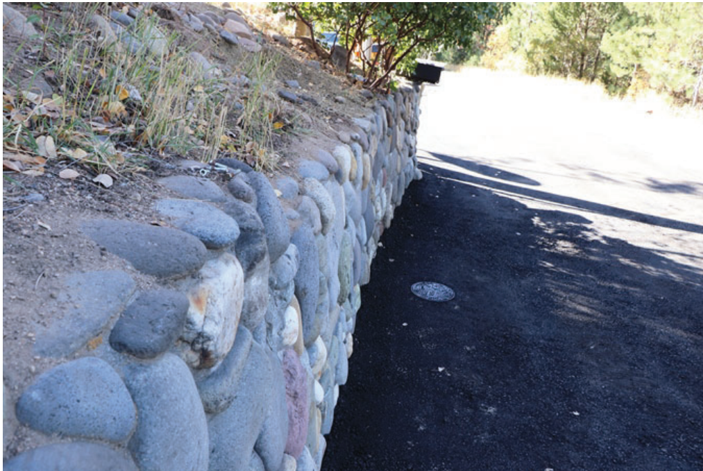
Photo 4: Another view of the subject retaining wall.
