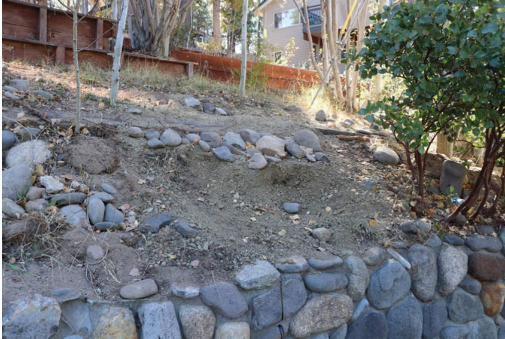
Photo 7: Area behind subject retaining wall that evidenced recent excavation.
