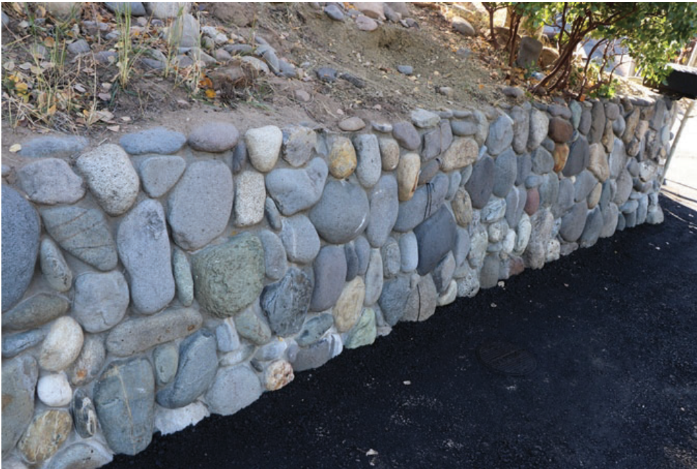
Photo 2: Closer view of the subject retaining wall.
