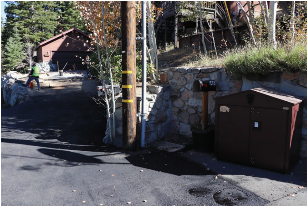
Photo 10: View of the area where the neighbor's retaining wall joins the claimant's retaining wall.
