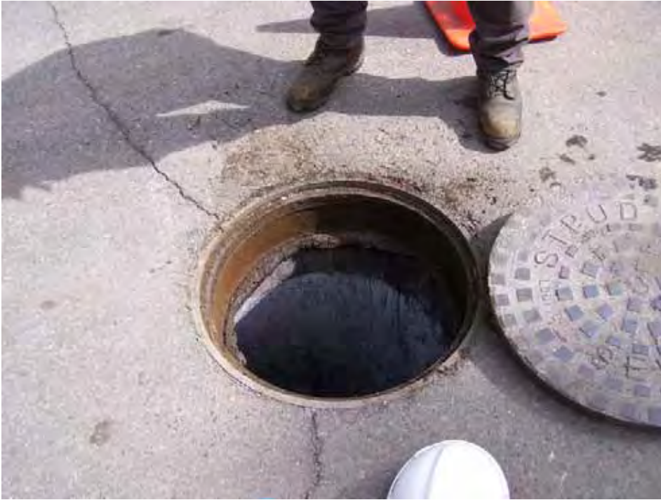
Description: Replaced MH Cover
