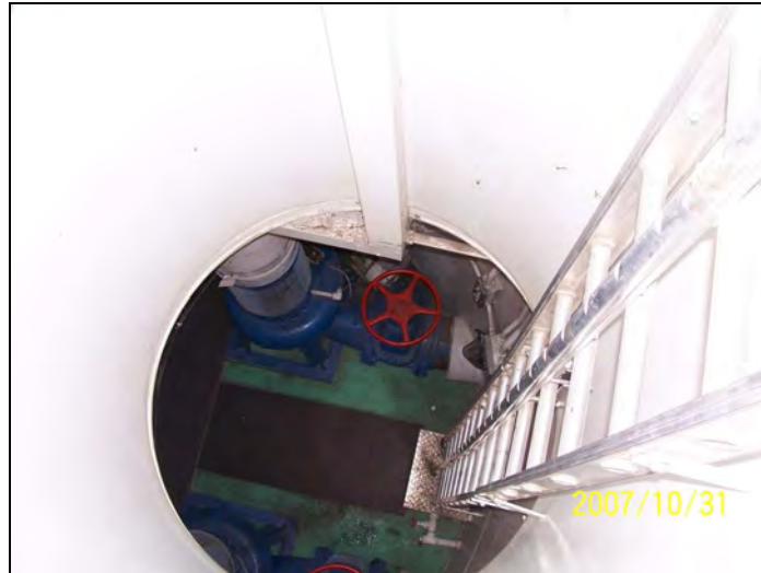
Figure 4-2. Ladder Access into Dry Well
