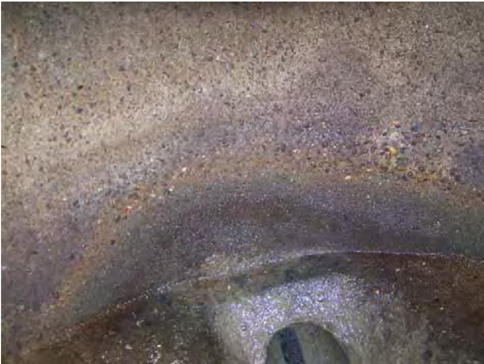
Description: Unlined Concrete – No corrosion
