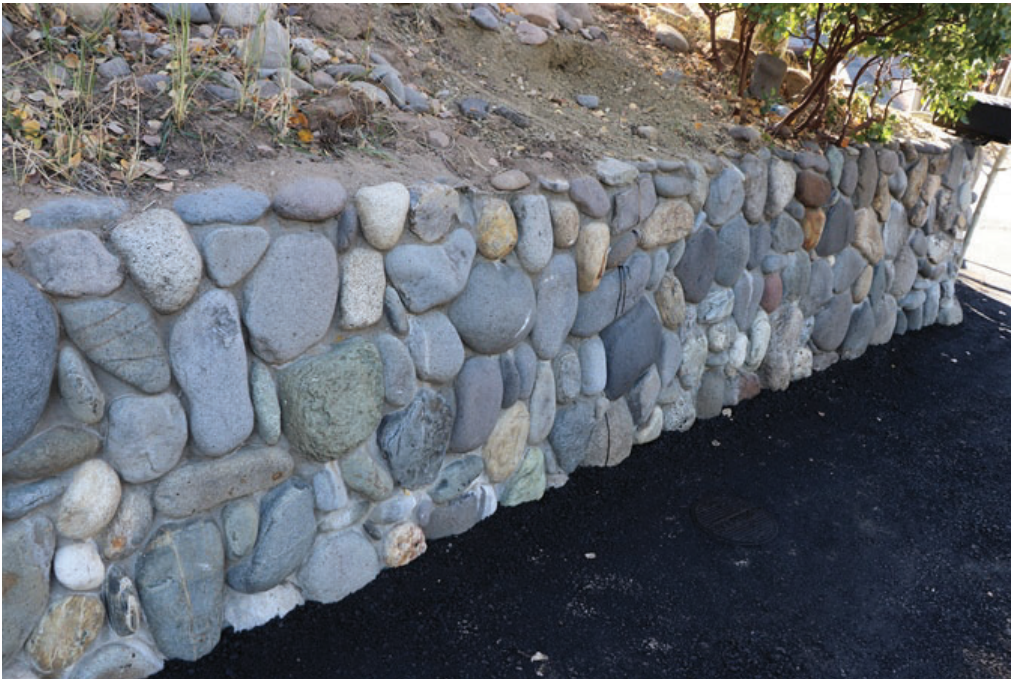
Photo 2: Closer view of the subject retaining wall.
