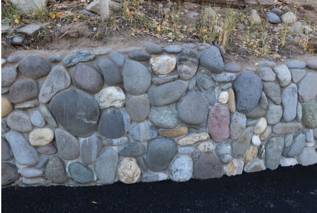
Photo 3: Another view of the subject retaining wall.
