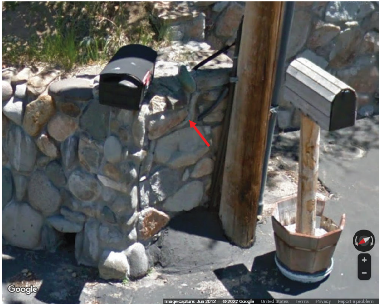
Photo 13: Google Street View Image dated June 2012. Note wall crack is evident in image.
