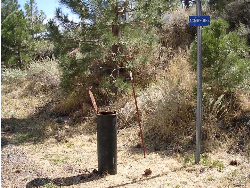
Photo of ACMW-01BE with no bollards and concrete pad for protection
