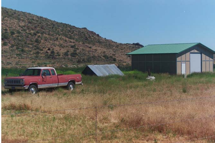
Figure 3. GW-04: Septic tank and leach field.
