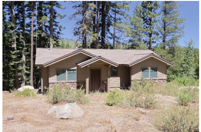
Figure 2 Grizzly Mountain Booster Station
