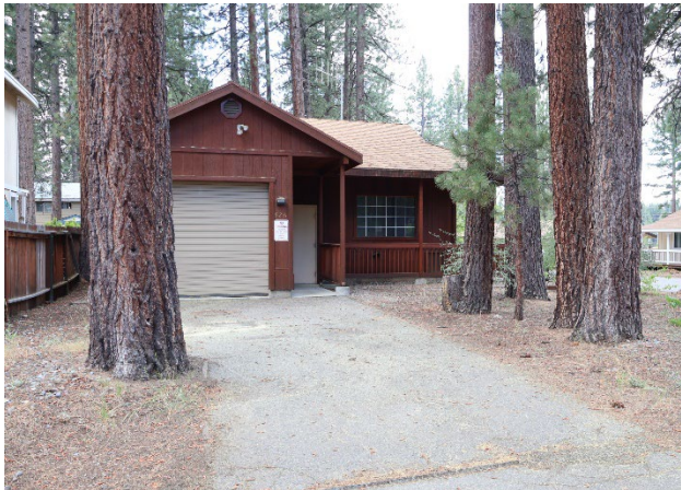
Figure 1 Paloma Well House
