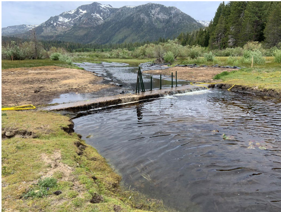
Figure 1. Site Conditions on June 20, 2022.
