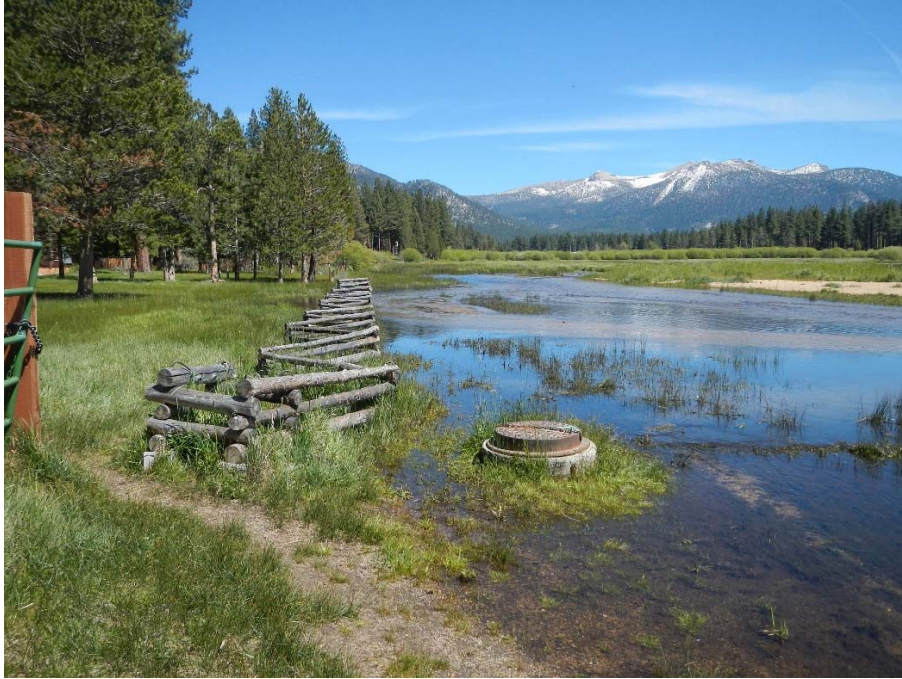
Figure 2-4. Inundation of the sewer easement near Bellevue Avenue at a flow of approximately 40 cfs, looking upstream, 20 May 2013
