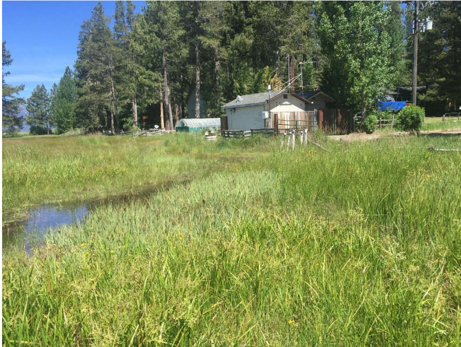
Easement Near Bellevue Pump Station (white stakes are at MH BV17)
