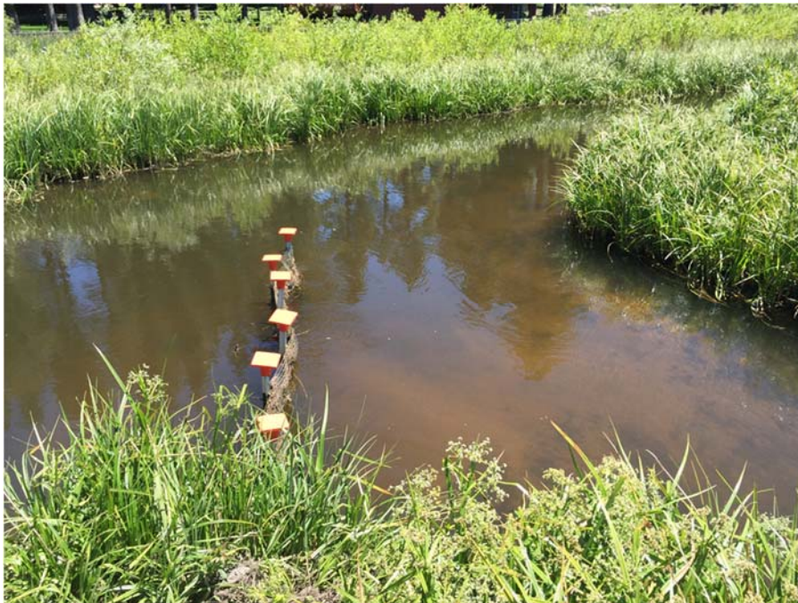
Figure 4-2. PC-3 flow diverter at head of PC-3; flow in PC-3 is towards lower right of frame
