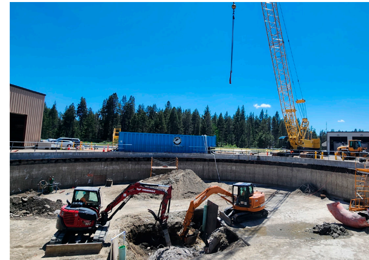
Repairing wastewater clarifier; installing a new water main; Tahoe Keys wastewater pump station upgrade
