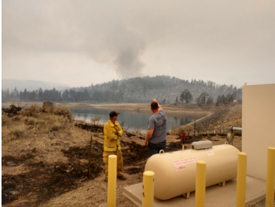
Pump Operator Buck McLelland and Water Reuse Lead Jason Glaze assess Tamarack Fire damage surrounding Harvey Place Reservoir.
