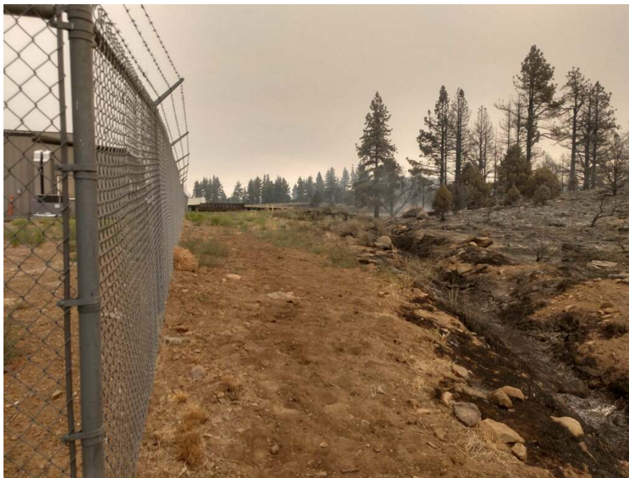
Fire break that protected District facilities during the Tamarack Fire
