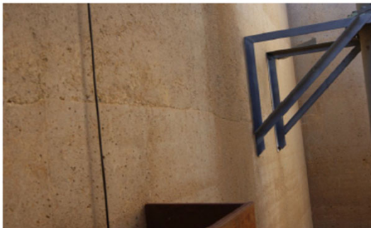
Figure 20 Emergency Pump Station - Horizontal crack of the vertical walls in the sump pit. Crack spans all 4 walls.
