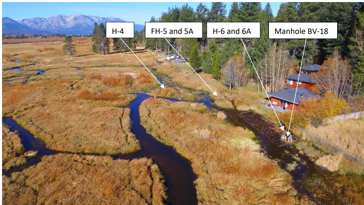
Figure 4-14. Upstream of Bellevue work area looking west, 14 Nov 2016 (with pilot channels diverting flow to left). District utility easement was inundated in area of BV-18 within overbank area right of the main channel of Trout Creek.
