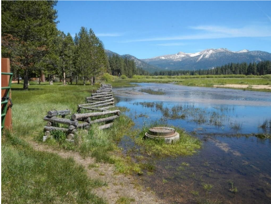
Figure 2-4. Inundation of the sewer easement near Bellevue Avenue at a flow of approximately 40 cfs, looking upstream, 20 May 2013.
