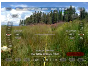
Road Fill Transect 2 Begin
