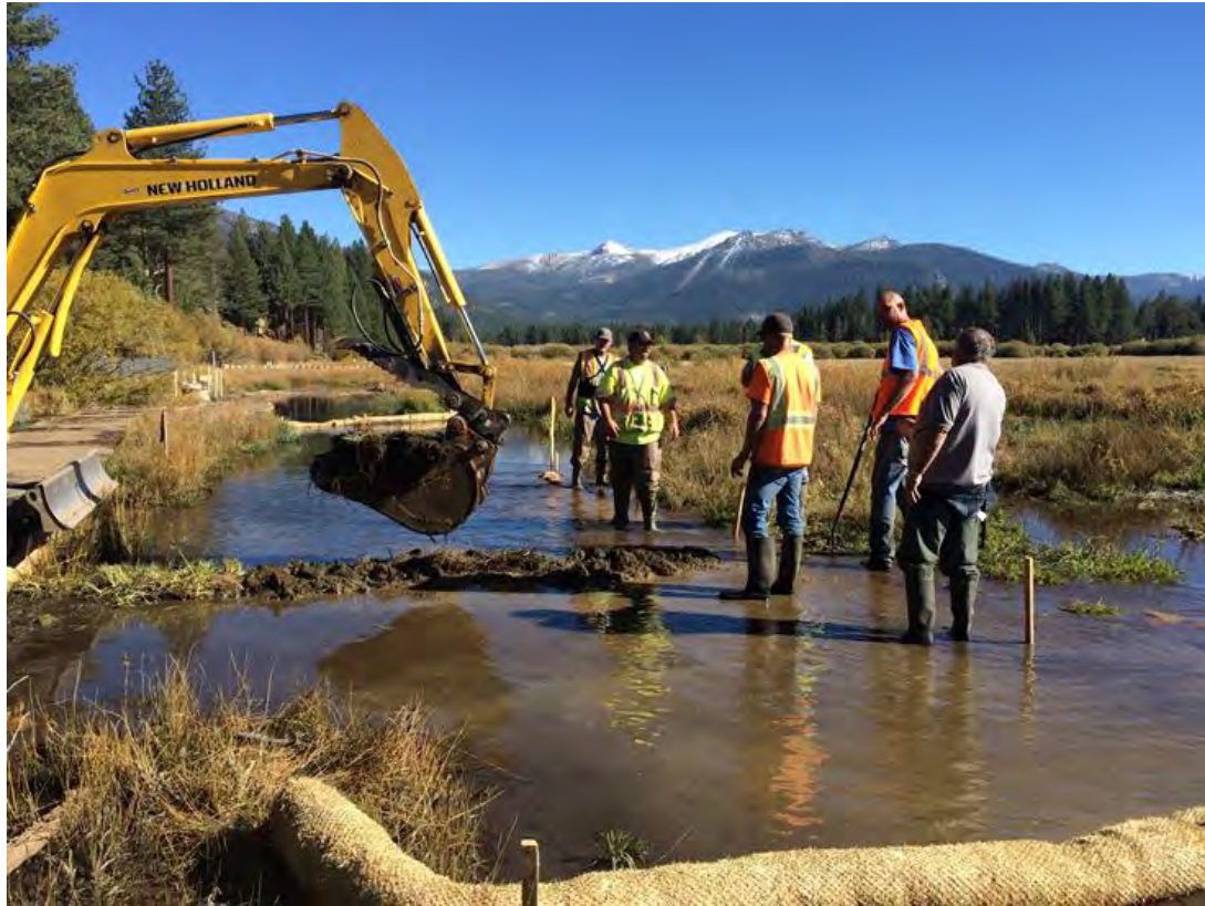
Photo 1. Construction of Hummock 4 looking south, October 6, 2014
