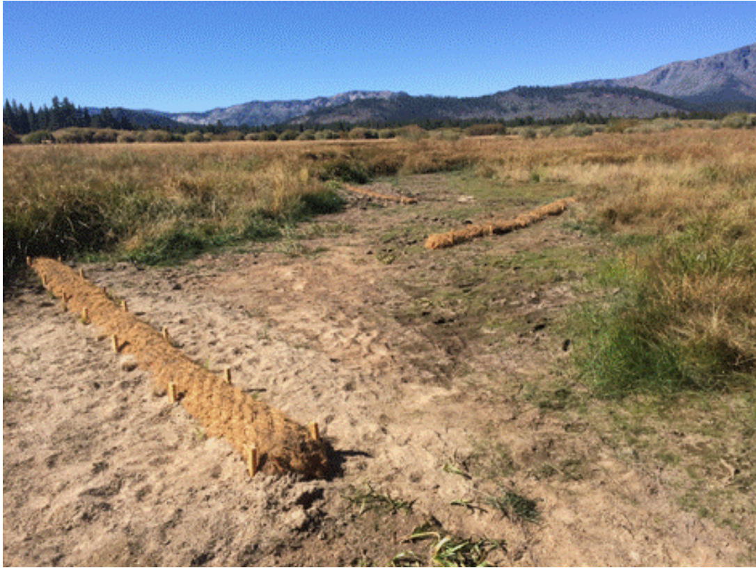
Photo 21. Coir log install year 2, September 17, 2015 near Hummock 1
