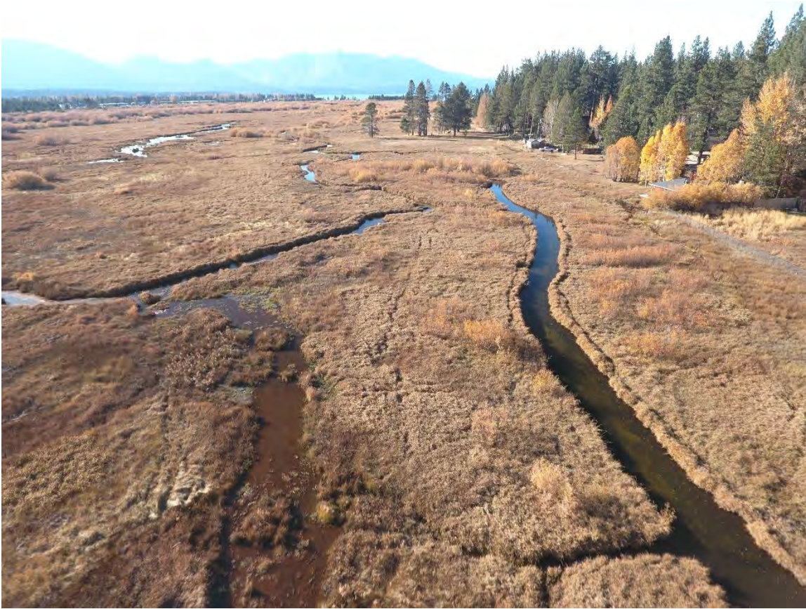
Oblique downstream view (3 of 8)
