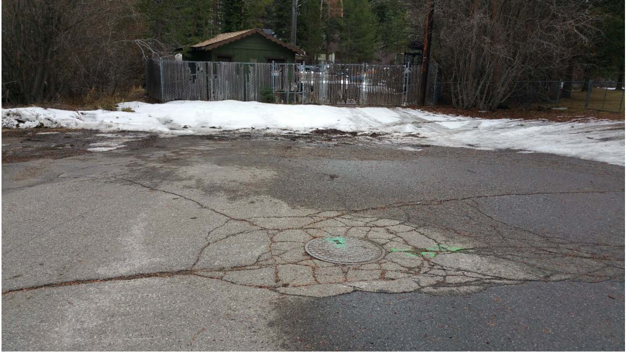
1. Sanitary sewer manhole and view of well house
