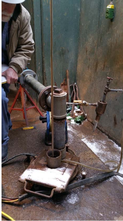
11. Pump discharge head and access pipe for spinner tool
