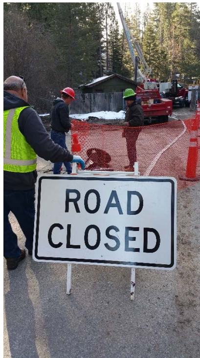
2. Traffic control and protection around sanitary sewer discharge to manhole
