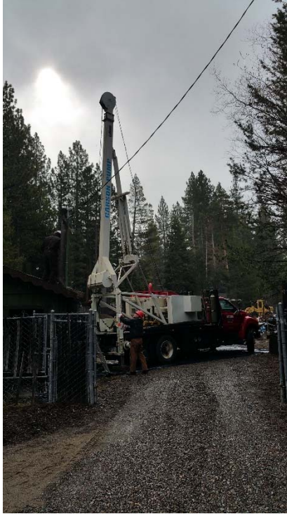
19. Carson Pump rig
