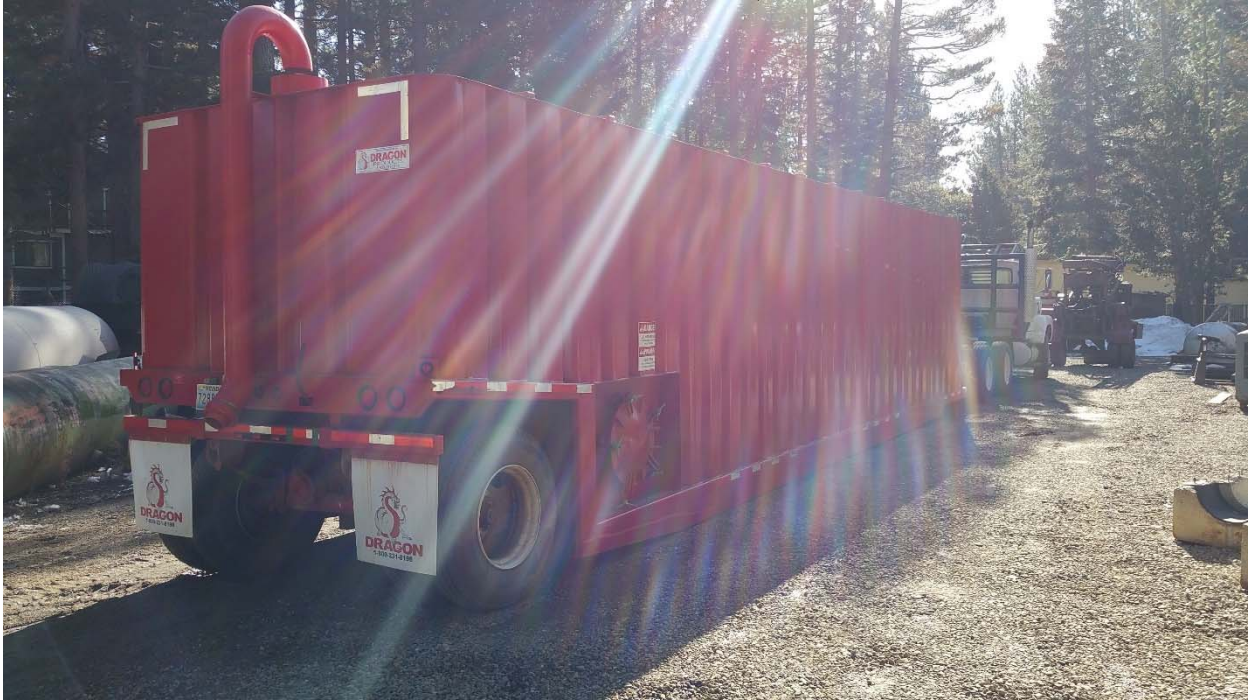
5. Frac Tank for storing water prior to discharge to sanitary sewer
