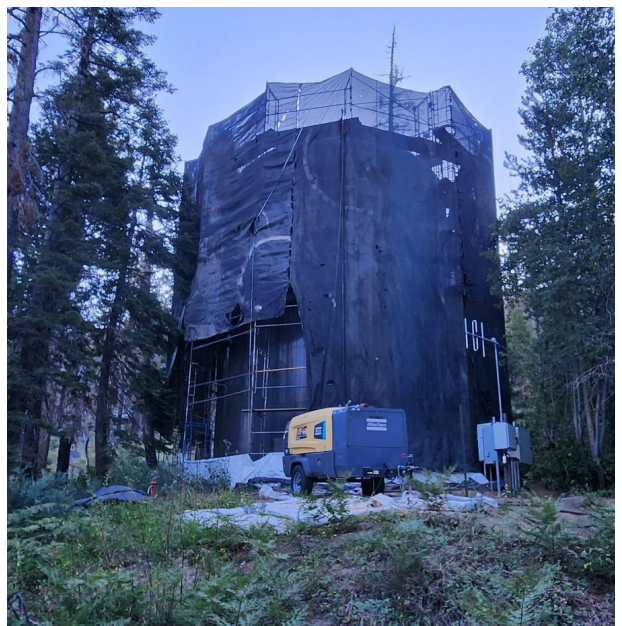
Recoating Christmas Valley water tank to extend its useful life.
