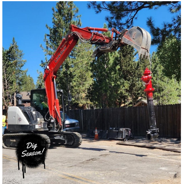
Upsizing waterlines and installing fire hydrants for community wide fire flow.
