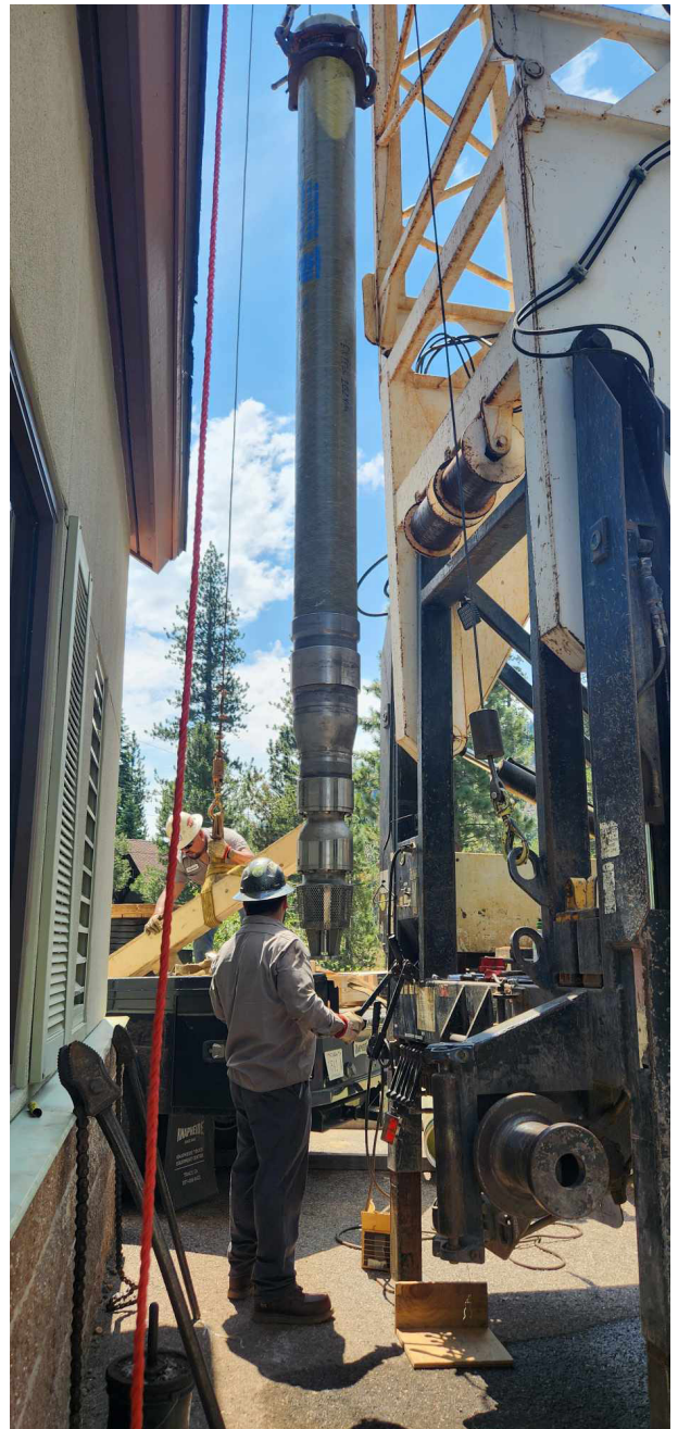
Rehabilitating South Upper Truckee well to provide high quality drinking water.
