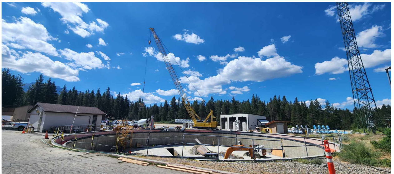
Replacing a secondary clarifier at the wastewater treatment plant.
