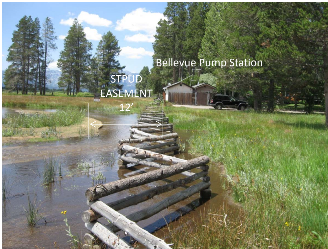
Figure 1-3. Looking west toward Bellevue Pump Station, July 2013.
