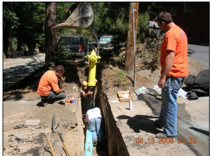
Installation of New Waterline in the Street (Photo courtesy of North Tahoe PUD)
