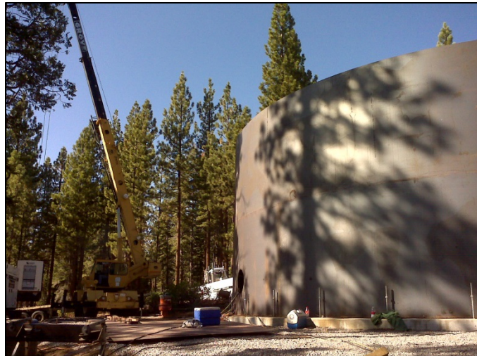
Tank Construction (Photo courtesy of North Tahoe PUD)
