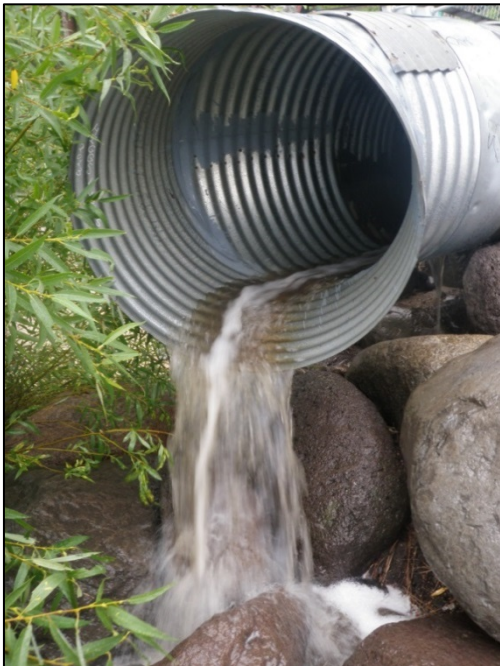
Storm Drain Outlet (Photo courtesy of Tahoe Resource Conservation District)
