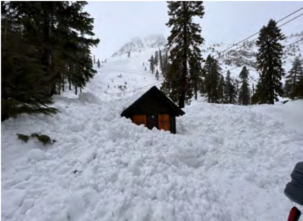
An avalanche at Fallen Leaf Lake took out power to three sewer pump stations.
