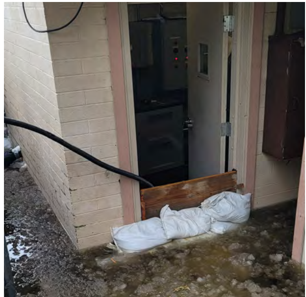
Temporary flood barriers and pumps were installed to reduce the amount of stormwater flowing into the sewer system.
