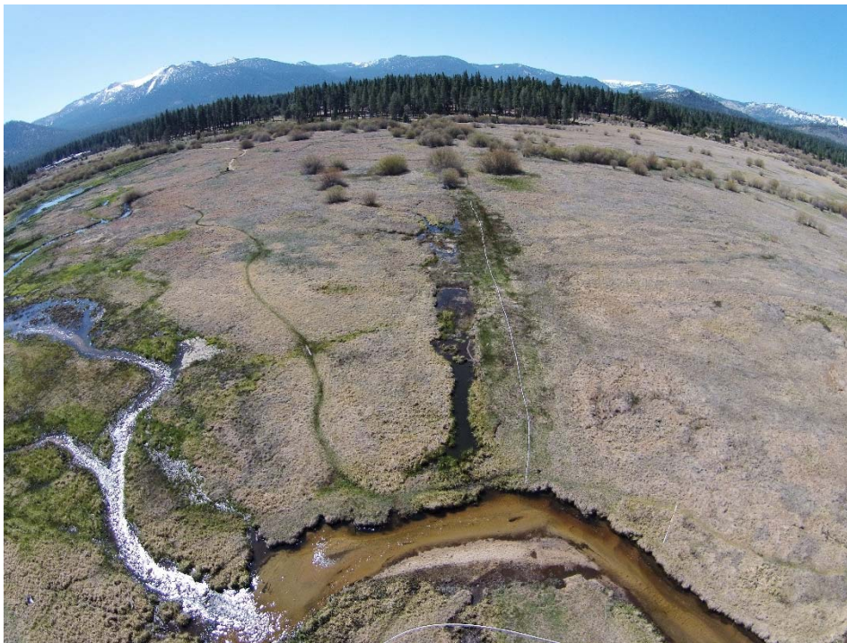
Figure 4-7. Aerial view of road fill removal area looking south, 17 Apr 2015 (road fill removal in right center of frame, pilot channel outlet in left foreground)
