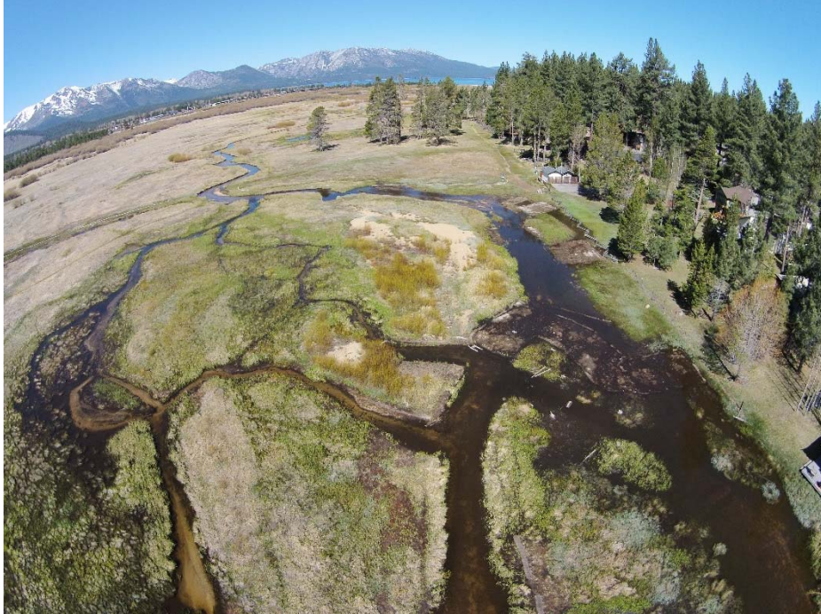
Figure 4-6. Easement and avulsed channel area looking west, 17 Apr 2015 (hummocks in right center of frame and along fence, pilot channels on left overbank)
