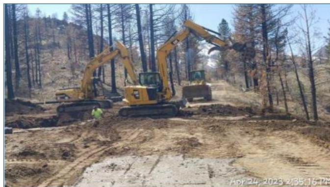
Dresser Ditch – Debris Removal from access road, erosion repairs, culvert restoration
