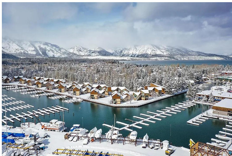
View of the Tahoe Keys in South Lake Tahoe after a winter storm.
