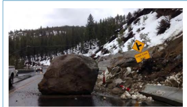
Extreme weather increases the risk of landslides damaging roads.
